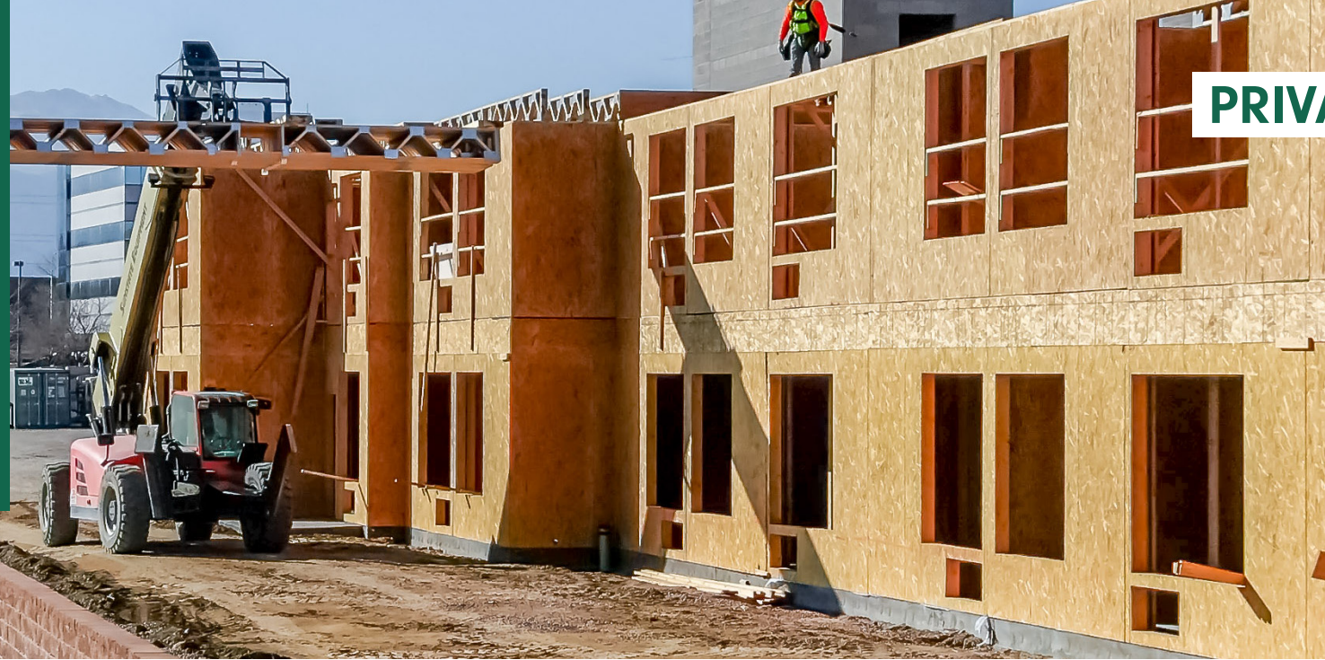
ACADEMY HEIGHTS 201 WORKFORCE UNITS - UNDER CONSTRUCTION
