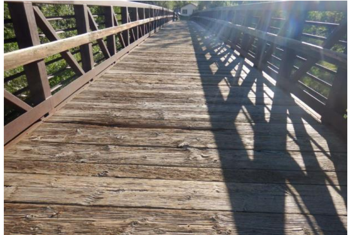
Current Decking for Replacement
