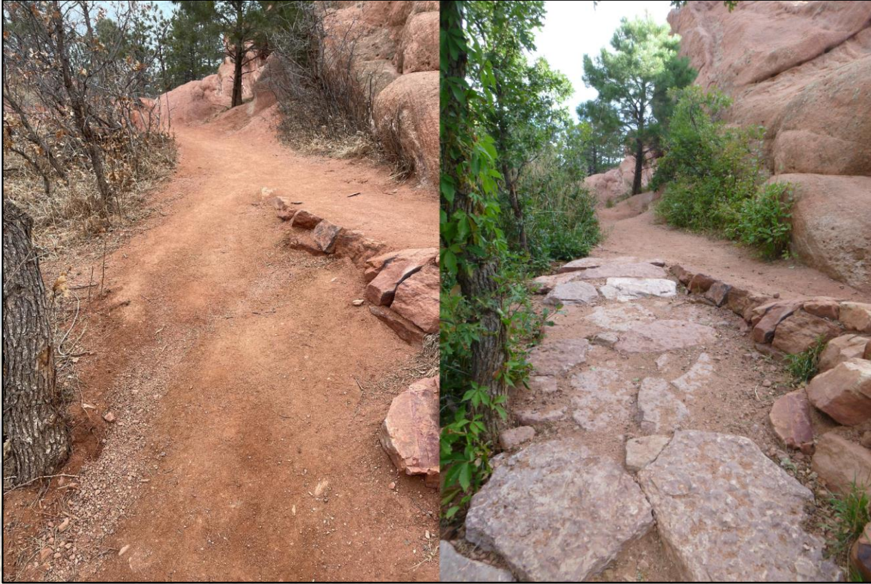
Rock armoring on Sand Canyon Trail
