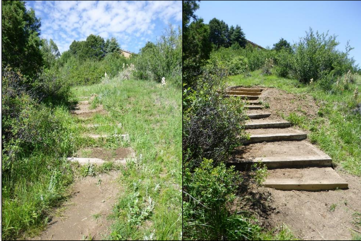
Timber step repair
