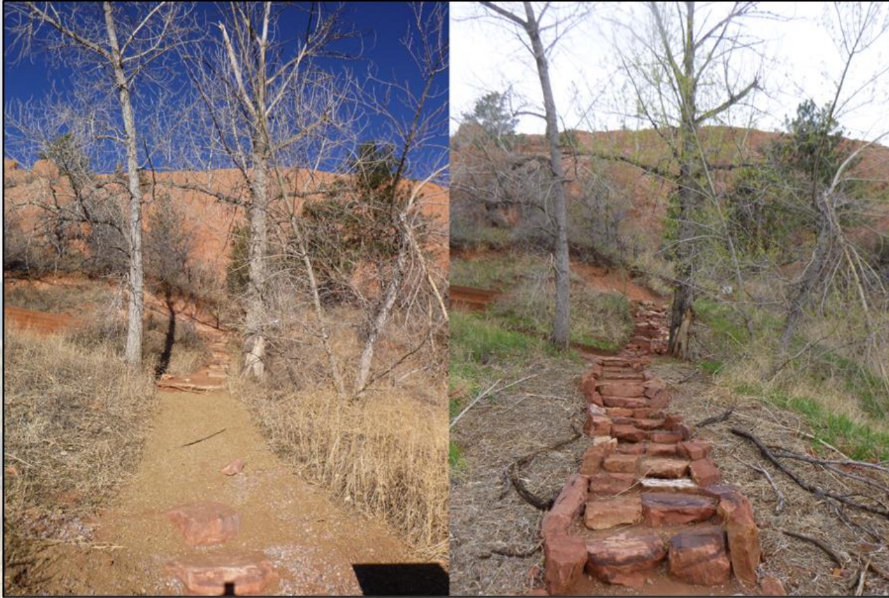
Rock Step Installation
