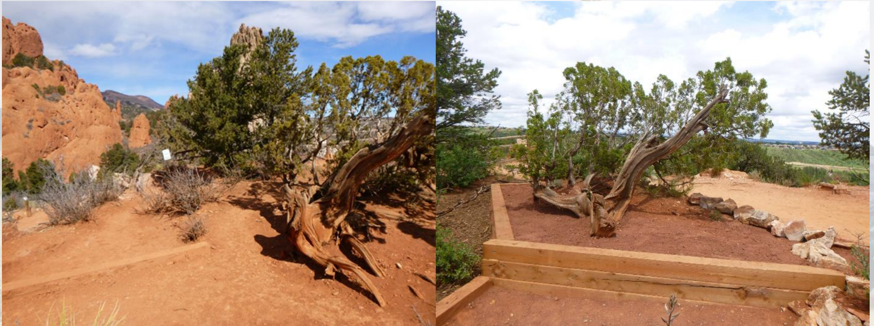
Timber and rock retaining structures near Ridge Trail
