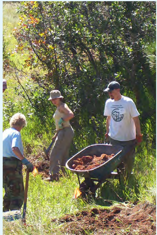
Volunteers lead by a trained crew participate in trail repair. Source: City of Colorado Springs
